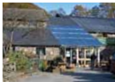
Staveley Wilf's Cafe Mill Yard Staveley LA8 9LR
